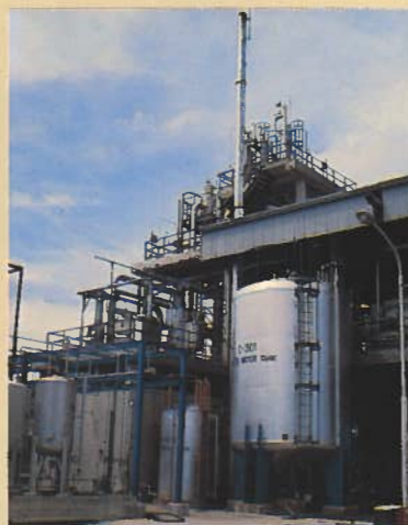
The first alcohol pilot plant from agricultural produce as alternative source of energy is an achievement of the cooperative project between TISTR and the Japanese Association of Industrial Fermentation. The application of innovative technology and sophisticated equipment facilitates energy saving process with the production of 99.5 v/v % ethanol suitable as gasoline substitute for automotive use.
