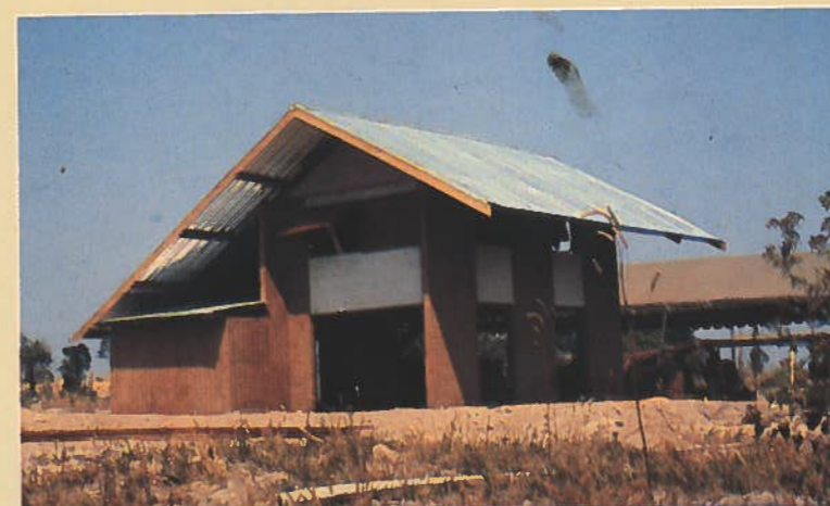
Soil-cement blocks for low-cost rural housing construction.
