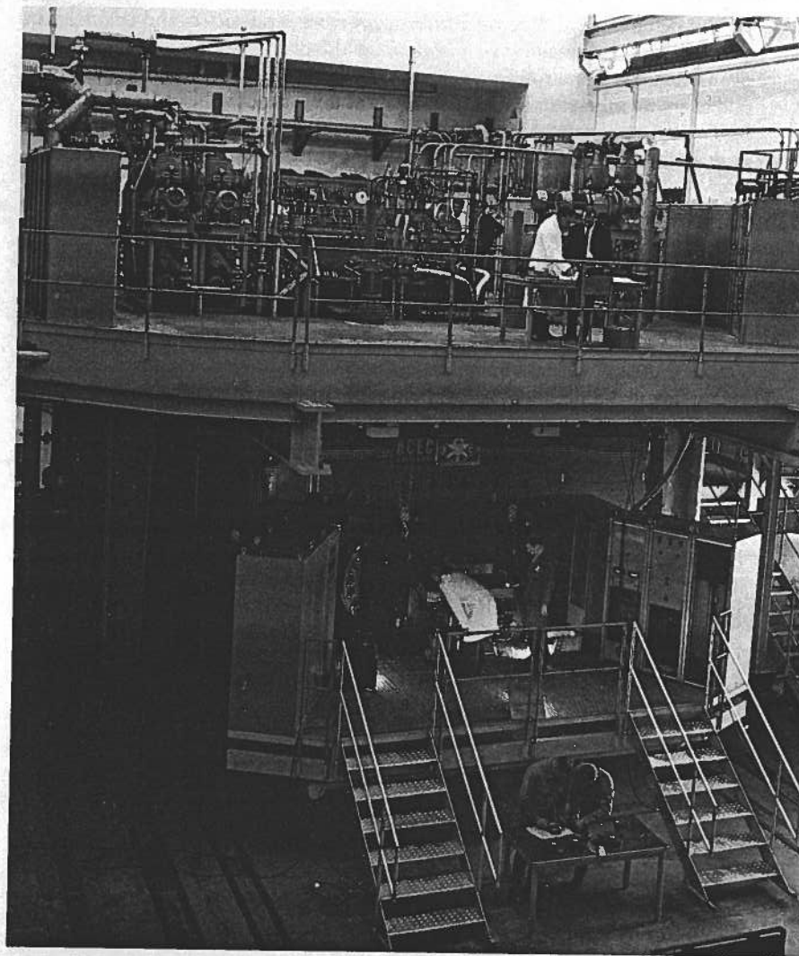
Fig. 3.2. European "perfectionism" vs. American "pragmatism." This is one of three giant, very sophisticated electrostatic separators built by CERN in the early 1960's to purify secondary particle beams. Brookhaven initially had similar grandiose plans, but opted for a simpler, more conventional device. CERN's decision meant that the laboratory was late to exploit the potential of its new proton synchrotron when it first worked, although in the years to follow it built some of the best separated beams in the world. Photo courtesy PHOTO CERN.
