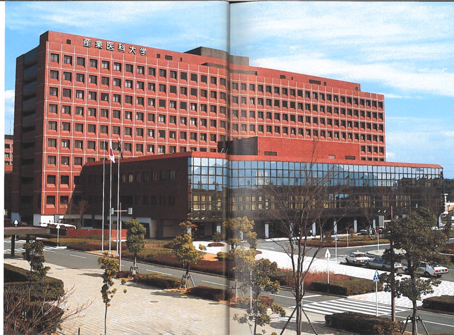
Full View of the University Hospital
