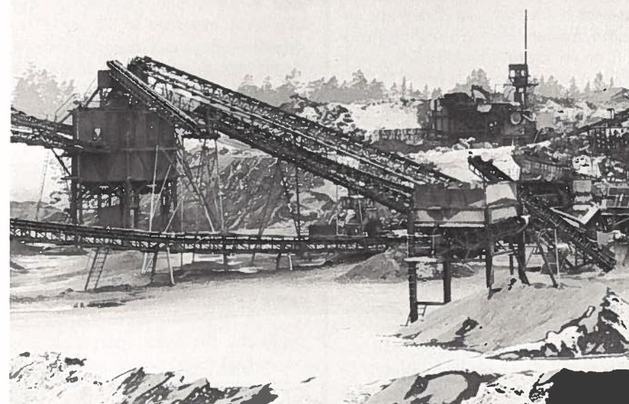
The limit values can be regarded as quantified minimum provisions on the work environment, and when planning new plants and processes they should be included in the specifications. A quarrying plant, above without moistening and below with moistening.
