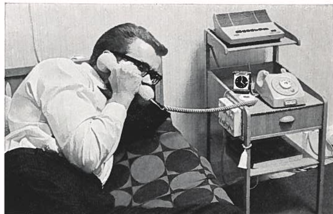
Communication is important. Radio and telephone for outside contacts, intercom for contact with service personnel and with the main entry. Switches for the lighting and an emergency signal are found at the bedside table. A smoke detector of fire is in the apartment.
