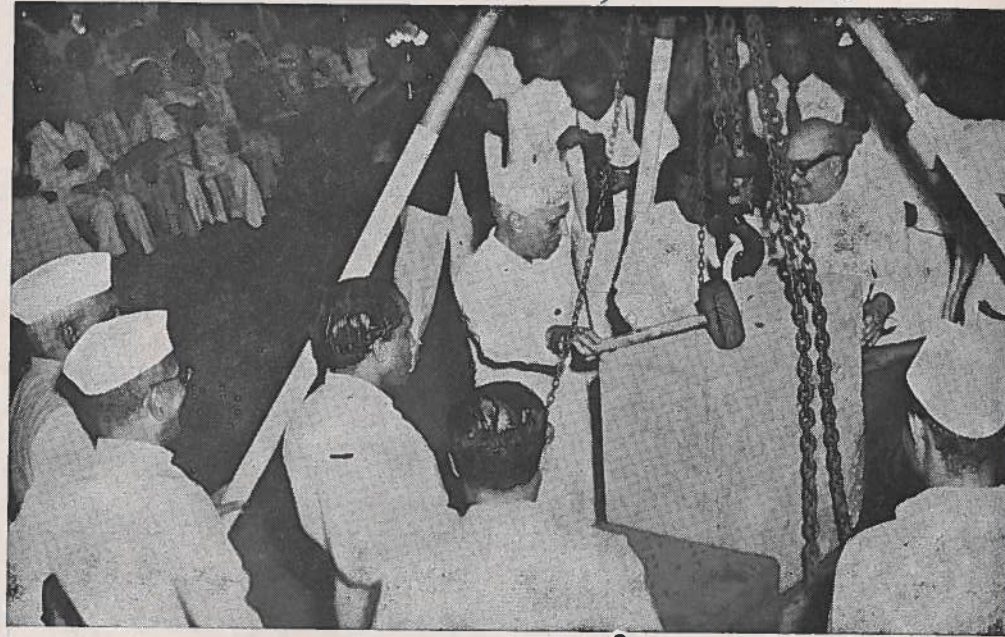
Late Prime Minister Jawaharlal Nehru laying the foundation stone for the Institute building
